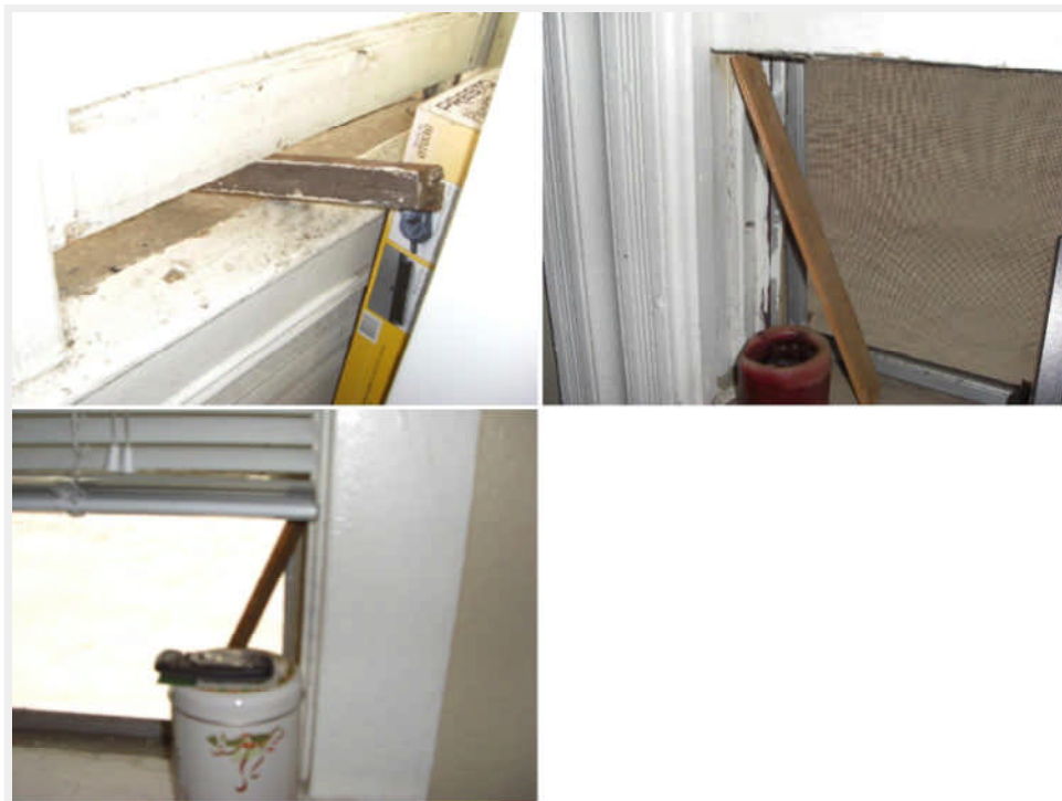
Counter balance and weights are broken in windows - Repairs needed.
