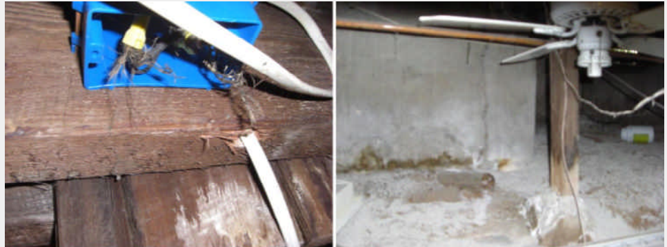
Open junction box with exposed wiring and a fan (not tested) in the crawl space.
