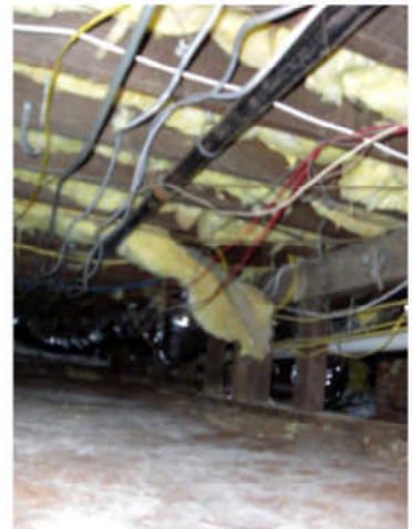
Open j-box and exposed wires hanging out, and insulation falling down.
