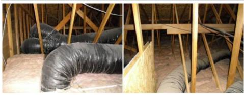
Return and Filter Fair. Filters need cleaning or changing in the near future. Excessive buildup of dirt in the air return duct behind the filter suggests cleaning of the cooling coils may be in
