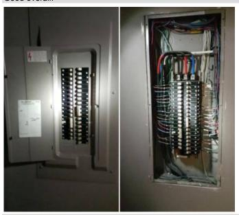
Circuit Breaker Sizing: Good overall. Wire Type: 100% copper. Wire Sizing: Good overall. Grounding: Unable to check without electricity. Outlets: Unable to check without electricity. Switches: Unable to check without electricity. Fixtures: Unable to check without electricity. A/C OPERATION: Unable to check without electricity. Unable to check without electricity. Heating System: Ductwork: Flex round, Appears serviceable. A/C Controls: Unable to check without electricity.
