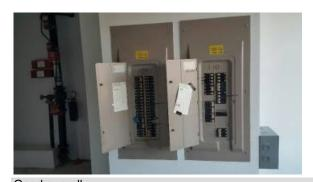
Circuit Breaker Sizing: Good overall. Wire Type: 100% copper.
